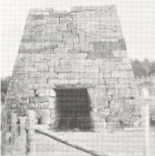
An old picture of Glenwood furnace. This stack is 38 feet high and was erected in 1849.
