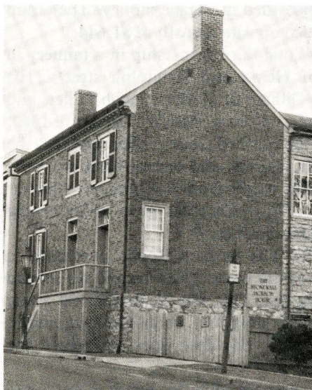
The restored Stonewall Jackson House in Lexington, 1981.
