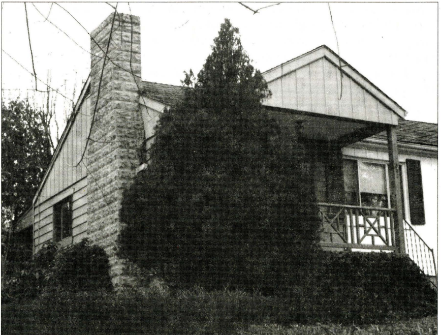
Below: Rockface block chimney on a Walker Street home, Lexington
