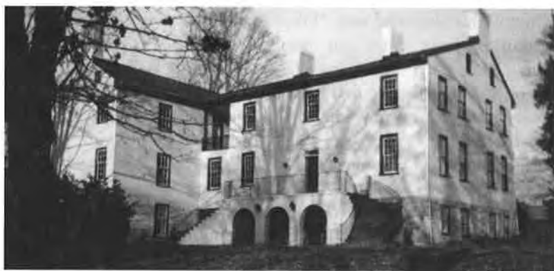
The main house of the former Sunnyside Dairy (now a part of the Kendal At Lexington retirement community).
