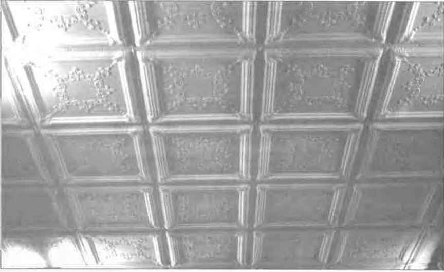
Figure 4. Pressed metal ceiling in store in downtown Lexington, Virginia. Photograph by author.
