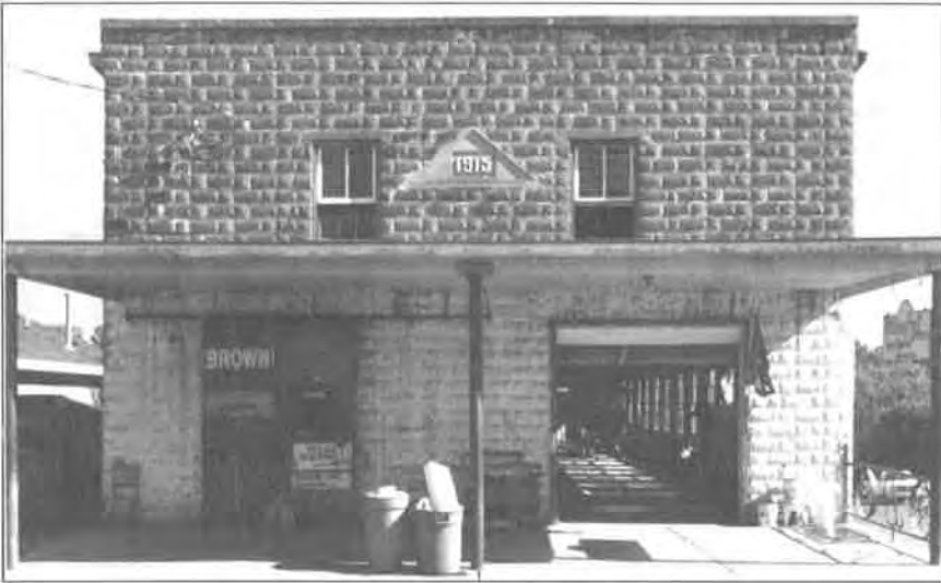
Figure 2. Frank Brown's rockface concrete-block blacksmith shop, 1915, Lexington, Virginia. Photograph by Delos Hughes.
