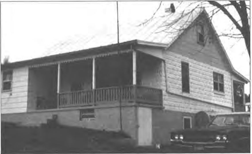
Figure 11. Charles Staton's ca. 1945, rockface concrete block house in the Kerrs Creek area, Rockbridge County, Virginia.
