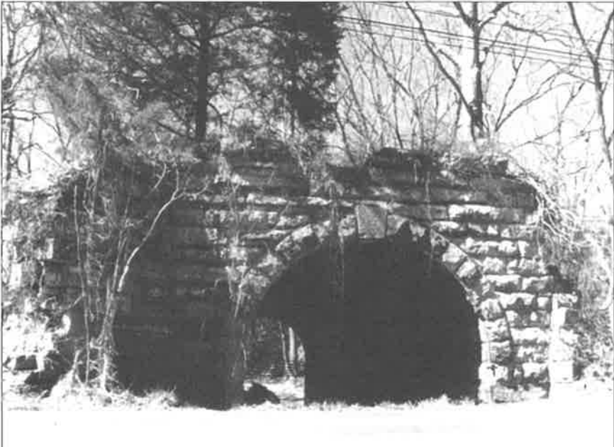
Below: Structure 3 (at 3590)—fourteen-foot arch on a tributary of Broad Creek.
