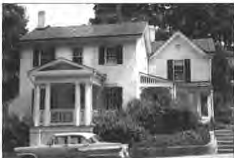
Left: The library building on August 5, 1965.
