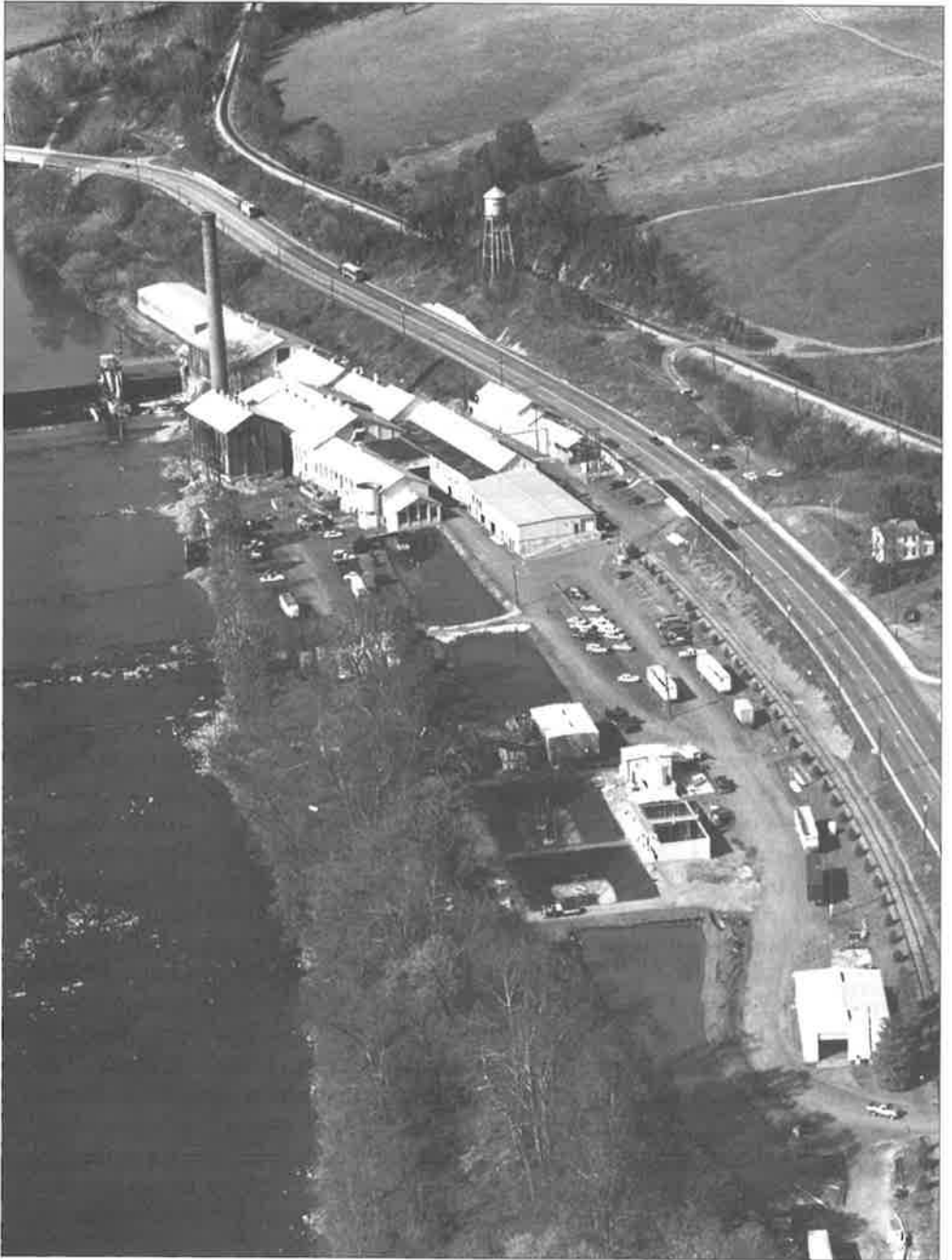
Bontex, Inc., plant on U.S. 60 in Buena Vista.
