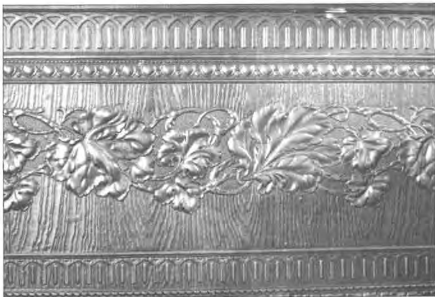
Figure 10. Imitation oak Lincrusta-Walton wainscoting from the 1912 Ogden House in Winston-Salem, North Carolina.
