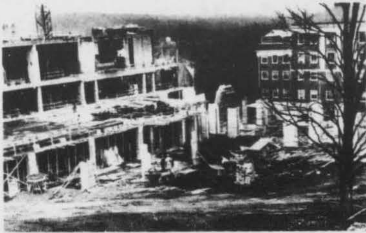
Construction progresses smoothly but new library holds surprises for students.
