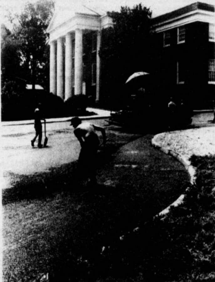
Workmen add finishing touches to a Commerce School driveway.
