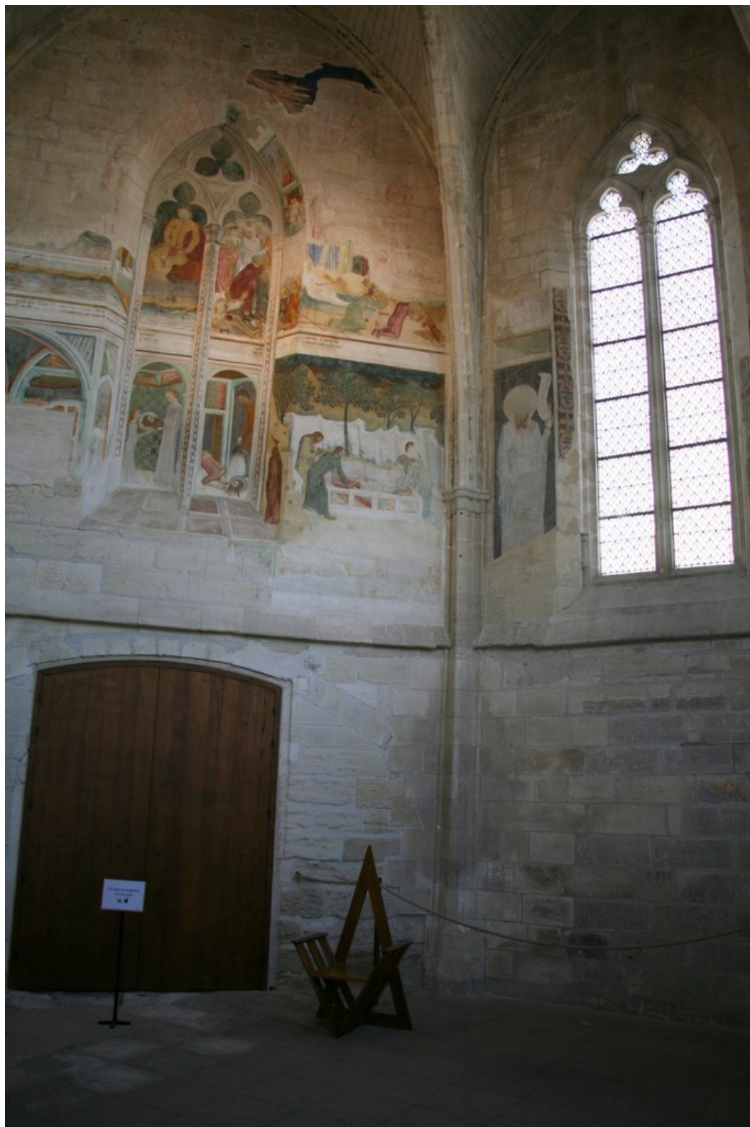
Figure 18: General view of the western wall of the Chapel of St. John the Baptist
