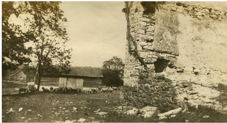
Ca. 1911 photo of Liberty Hall Ruins (foreground) and the 1799 Stable (center, mid). This photo of the stable, which doubled as a slave quarter, is the only known photo of building occupied by enslaved African Americans on Liberty Hall Farm.
