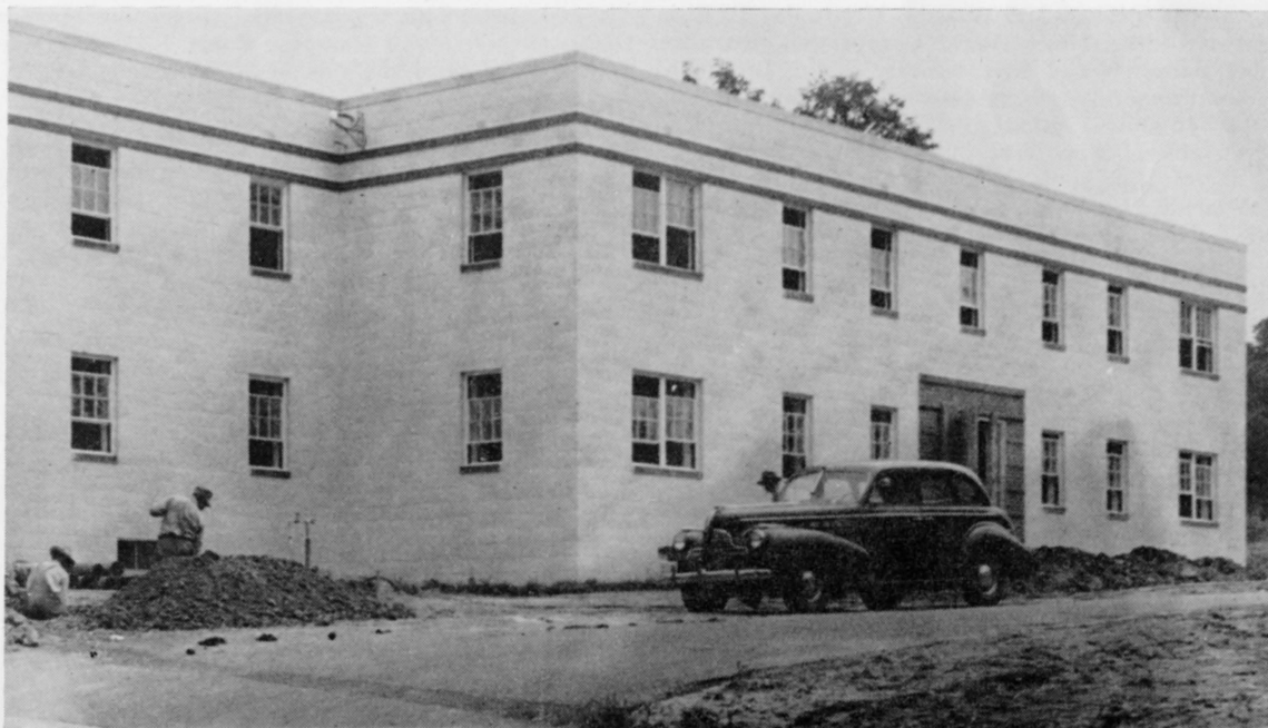
New Faculty Apartment Building
