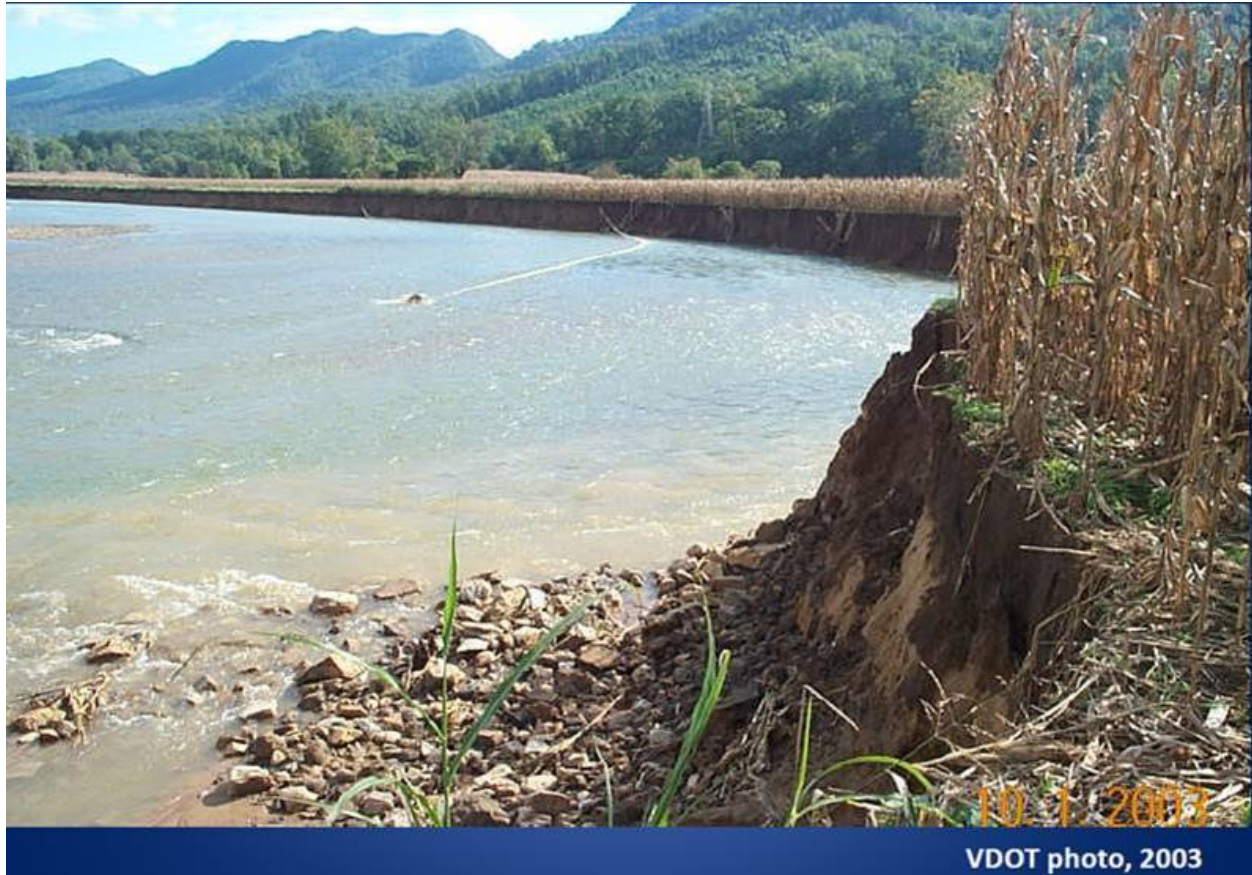
Figure 11. Severe bank erosion in 2003 on the Maury River (downstream of Jordan's Point) due to bar migration and growth following a dam removal in 1974 (photo credit: Virginia Department of Transportation).
