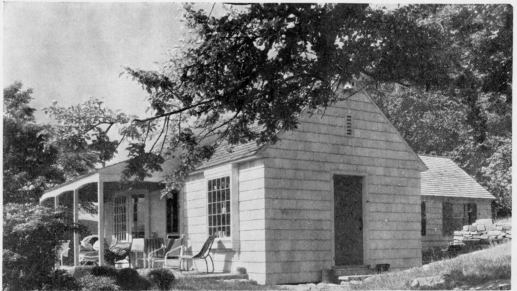
The porch across the front is arranged with a roof over but a portion of it; the flooring is flagstone.
