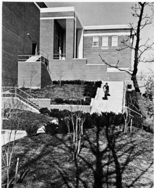
Addition to Doremus Gymnasium is another large project in the development program.
