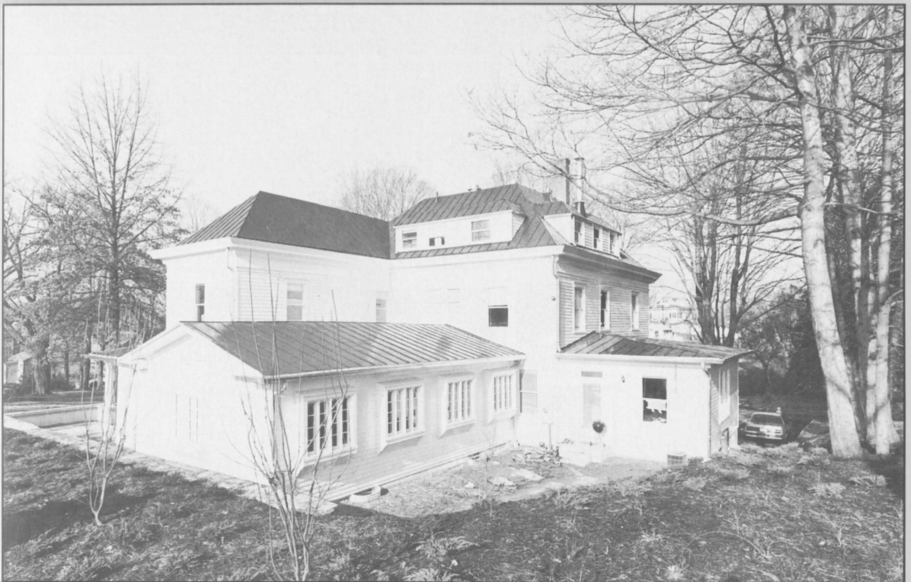
Fire escapes have been removed from the exterior of Sigma Nu (above), while an addition has been constructed to provide more space at Sigma Alpha Epsilon.
