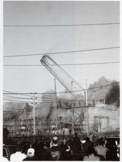
neatly in a self-contained pile of concrete and steel, thanks to a lot of planning—and 5,500 lbs. of explosives—on a clear Sunday morning in April.
