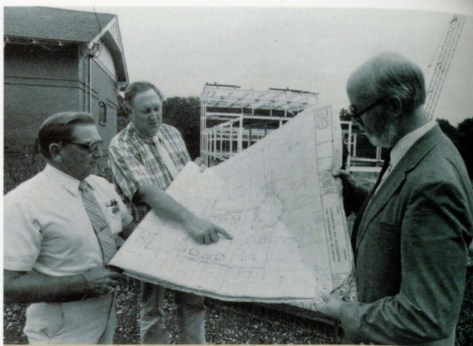
Parsons (right) reviews site plans for the Lenfest Center for the Performing Arts with Bill Wiseman (left), construction superintendent, and W&L's Scott Beebe, director of physical plant.
