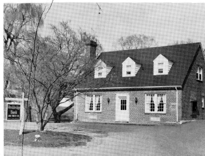
SOUTH MAIN BRANCH 708 South Main Street
